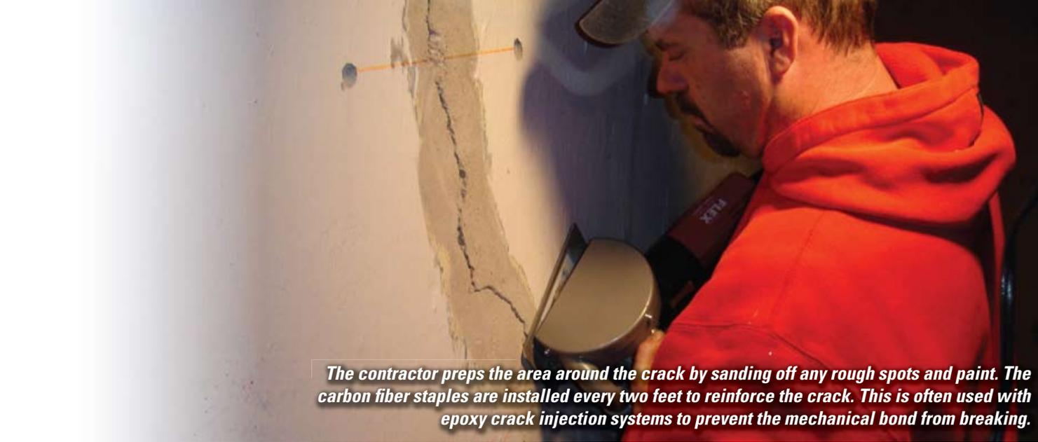
**The contractor preps the area around the crack by sanding off any rough spots and paint. The carbon fiber staples are installed every two feet to reinforce the crack. This is often used with epoxy crack injection systems to prevent the mechanical bond from breaking.**
