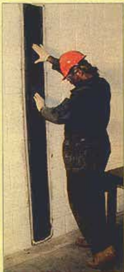
Figure 1. Applying vertical strap to reinforce masonry wall.
